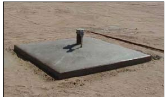
Example of a properly protected wellhead.
