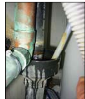
PVB with bolted in rubber plug
