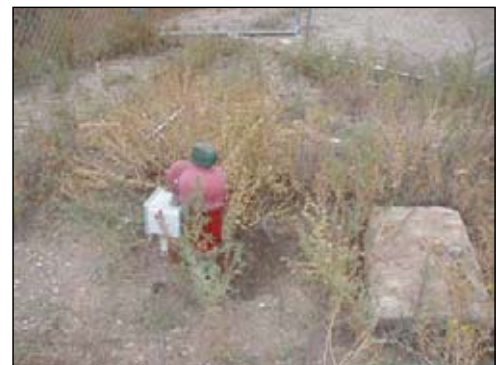
Another example of an unprotected wellhead.
