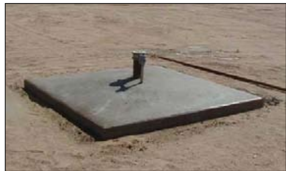
Example of a properly protected wellhead.
