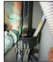
PVB with bolted in rubber plug
