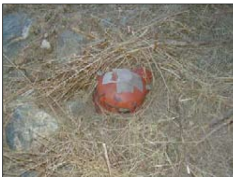
Example of an unprotected wellhead.
