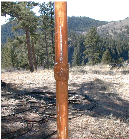
Iron bacterial slime on metal pipe joints.
