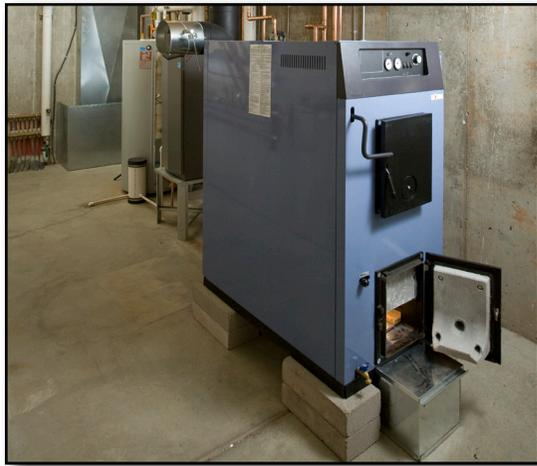
This TARM Solo 60 Mark II, 198,000 BTU/hour wood boiler is the heart of the system. It is one of the cleanest burning boilers on the US market. Bioheat USA, who has been importing TARM boilers from Denmark for more than 30-years, is introducing new boilers featuring real-time electronically managed combustion this year, further raising the bar on air emissions.
