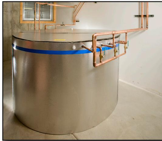
Integral to the system design, this 900 gallon water-filled thermal energy storage tank stores heat from the boiler. You stoke the boiler when it is convenient, the building uses the heat when it is needed.
