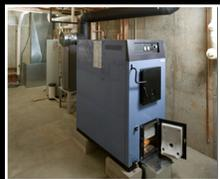
Manual fuel (wood) loading makes these systems very simple. With few moving parts, these systems are reliable and relatively inexpensive.
