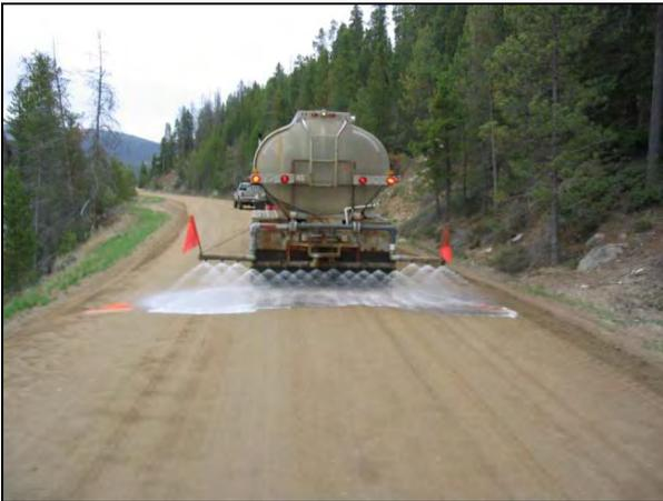
Figure 6.32. Magnesium chloride-based dust suppression product application.
