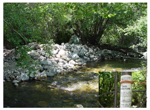
Photo 9. The diversion structure which is forcing water from the historic south channel of Cottonwood Creek into its north channel and the decree from the State of Colorado Division of Water Resources noting the closure of the structure on 22 May 2005 (insert).
