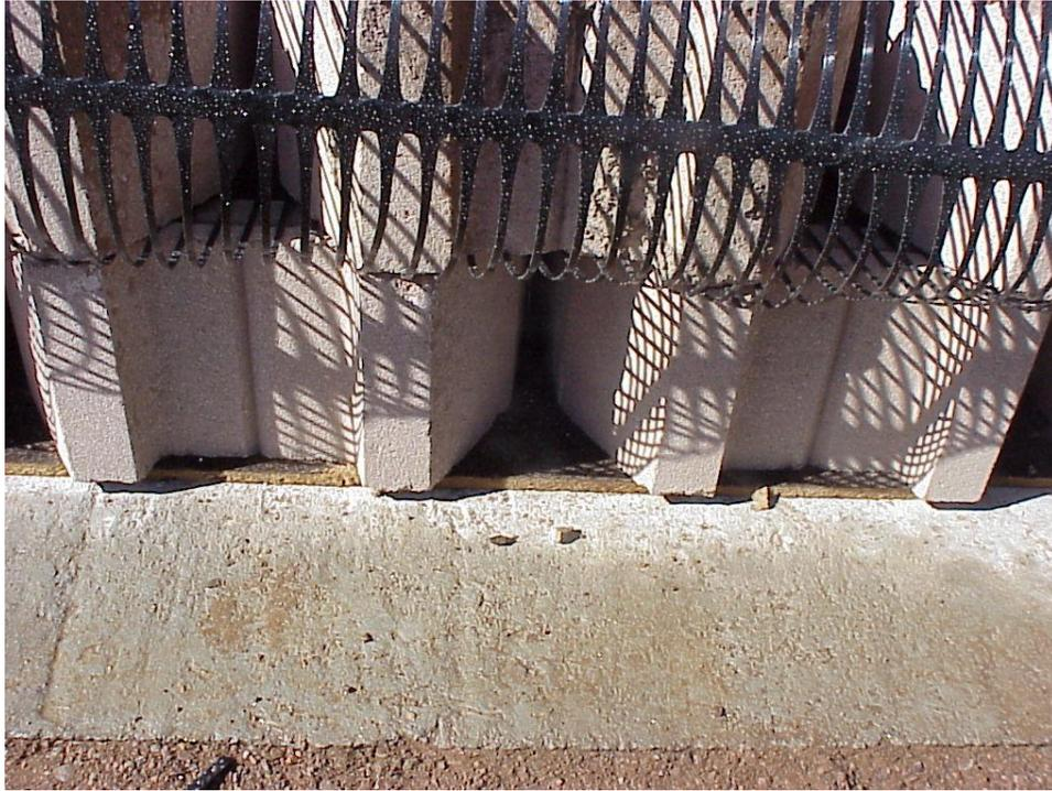
**Figure B-13. Expansion joint material was placed between the leveling bed and the first row of blocks.**
