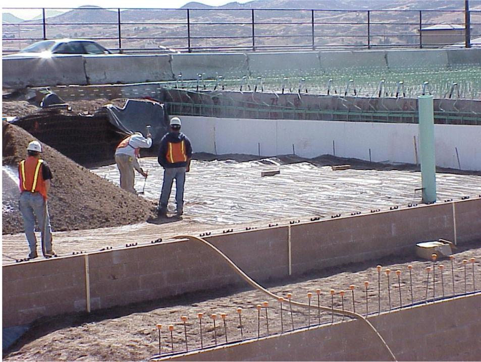
**Figure B-35. After the girders were placed, 75 mm sheets of low-density expanded polystyrene were placed against the back of the abutment wall. The area in the foreground between the lower and upper MSE walls will be covered with a membrane and paved with concrete (referred to as slope paving in Fig. 40).**
