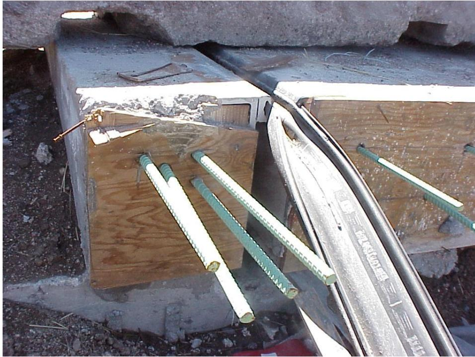
**Figure B-43. The approach expansion device placed between the sleeper foundation and approach slab.**
