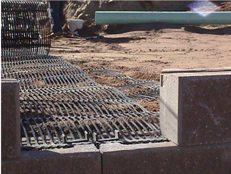
**Figure B-11. The facing blocks are fastened to the geogrid by the use of Mesa Standard Connectors which fit into the grooves of the blocks.**
