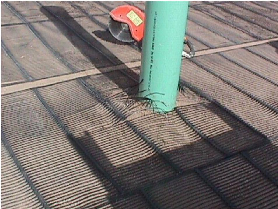
**Figure B-24. The geogrid was cut to fit over a drain pipe that went down through the middle of the structure. The pieces of geogrid were offset from one layer to the next so the longitudinal joints did not line up vertically.**
