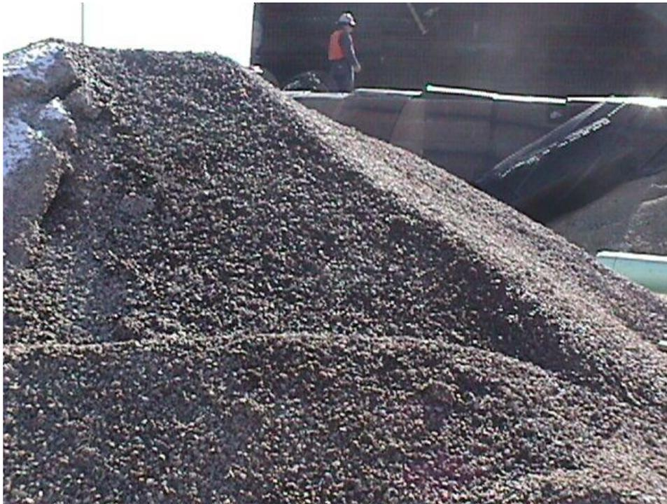
**Figure B-6. The 19 mm maximum size crushed stone aggregate used to fill in and for .3 m behind the blocks to facilitate compaction and drainage behind the blocks, prevent washout of the fines in the fill material, and facilitate compaction behind the facing.**
