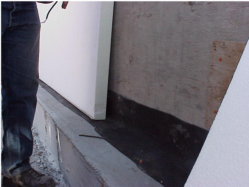
**Figure B-34. A plastic sheet was placed between bridge abutment and bridge foundation to facilitate water drainage.**
