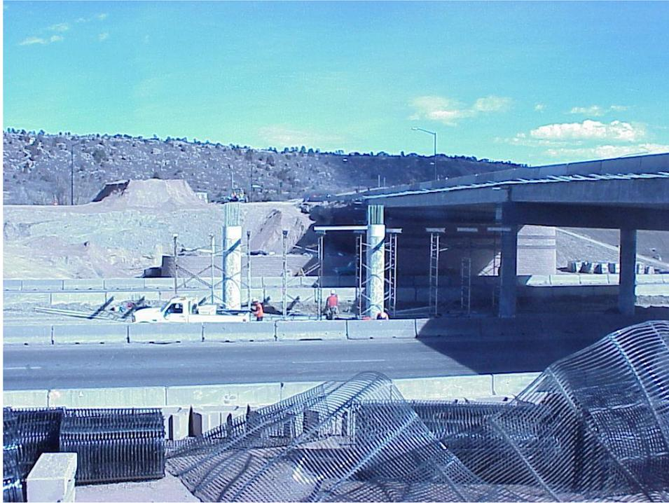
**Figure B-7. Rolls of Tensar UX 6 geogrid placed below the bridge foundation.**
