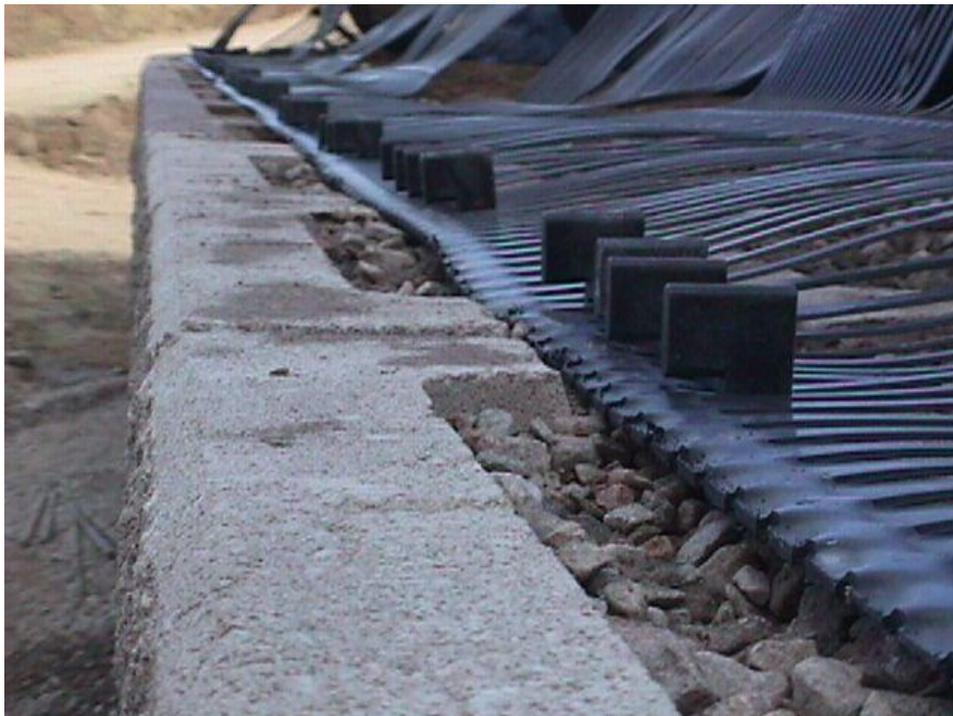
**Figure B-12. The rear of the block (to the right of the picture under the geogrid) is lower than than the front to allow for the thickness of the grid.**
